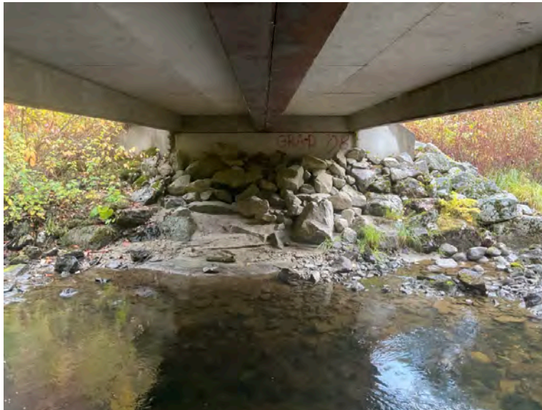
Right Bank Abutment when facing downstream
