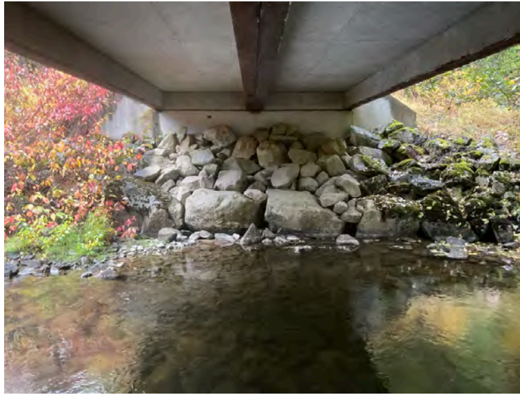
Left Bank Abutment when facing downstream
